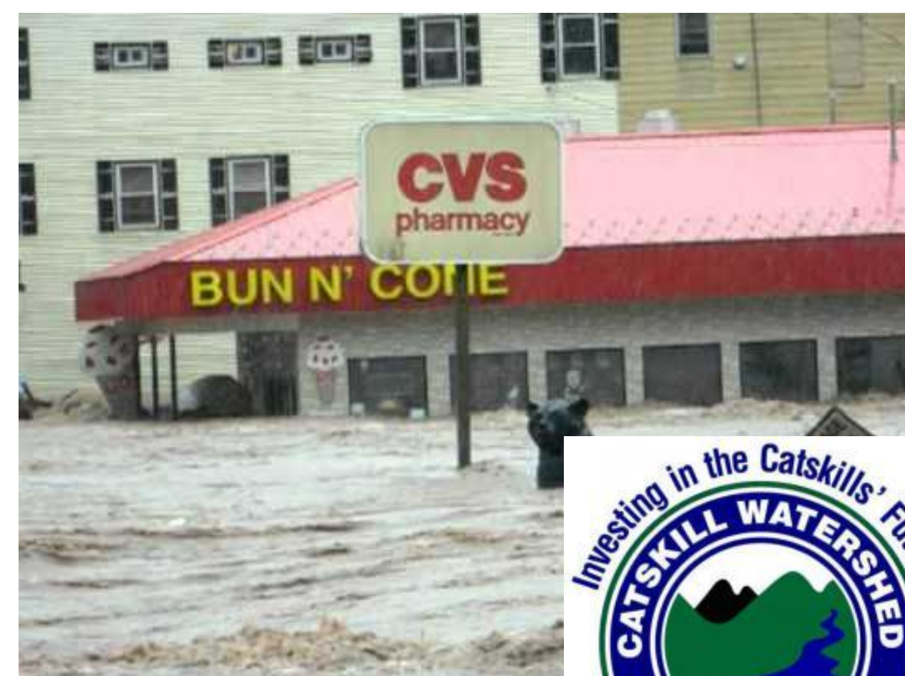
2011 flooding in Margaretville, NY
