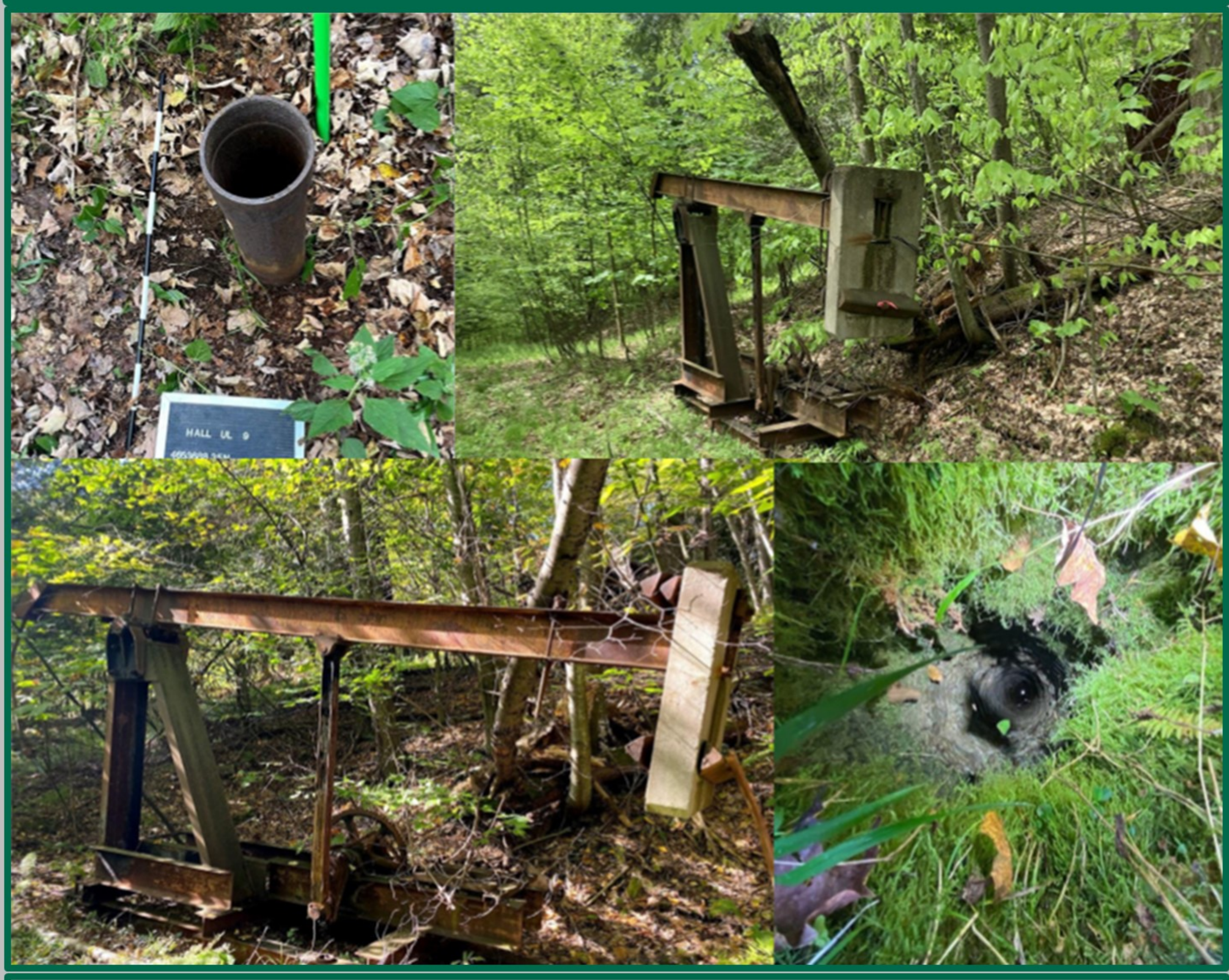
Image Set: Contains examples of both cased and uncased wells, as well as two pump jacks
