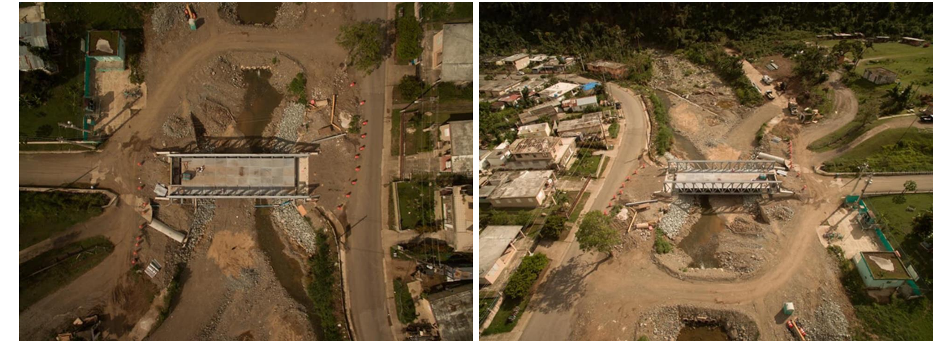
Figure 4 and 5. Seven Months Under Construction.
