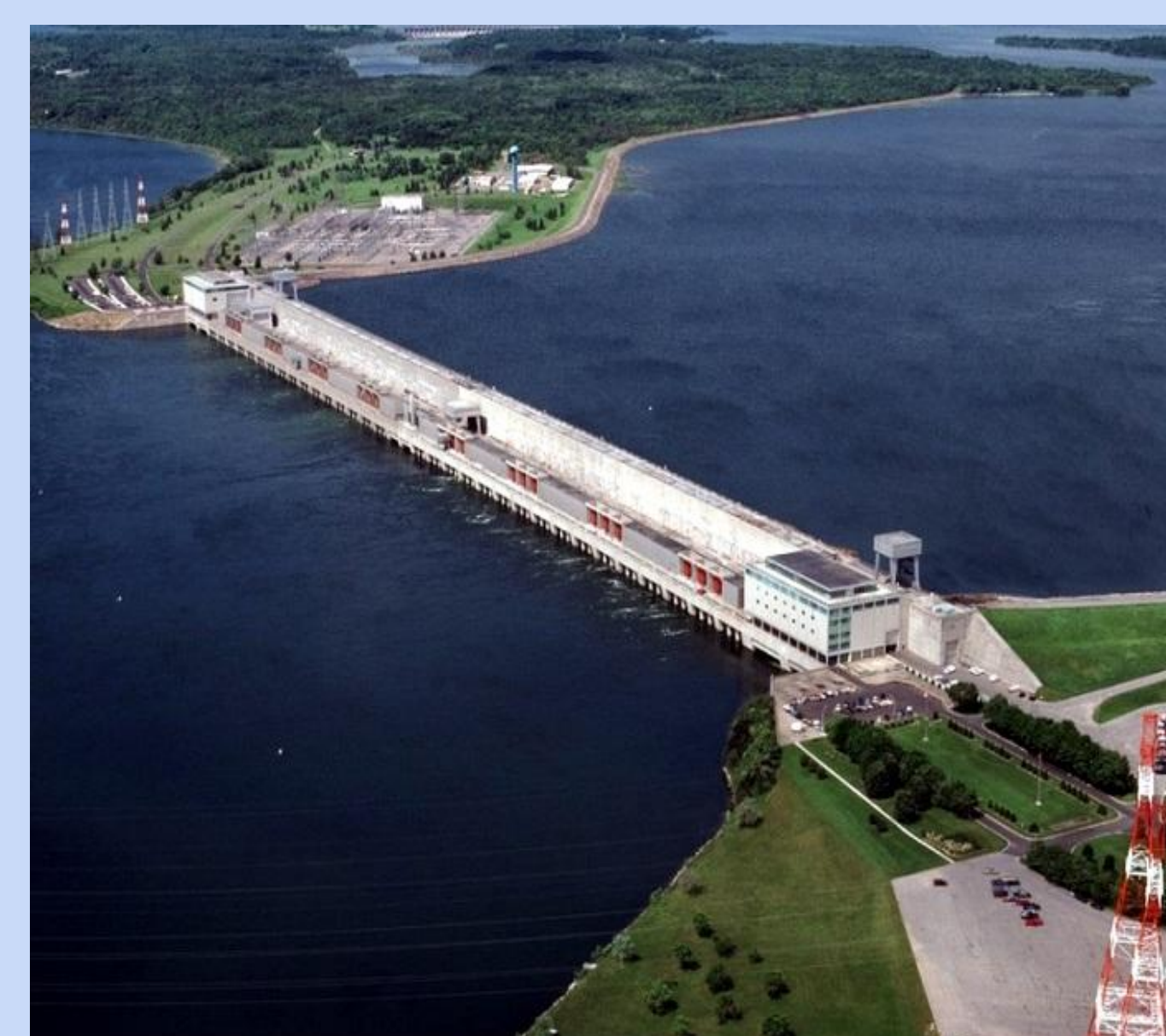
The Moses Saunders dam, located in Massena, NY regulates outflows of Lake Ontario (IJC.org)
