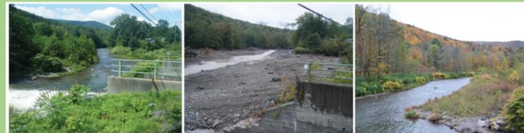
Esopus Creek at the Shandaken Tunnel outlet before (left) and after (center) the 2011 Hurricane Irene flood (photos from NYDEP). The right photo (courtesy of P. Knuepfer) shows the same site in October 2019. Note the stabilization of channel is now left of pre-flood position. Also note the revegetation of the rightmost bank in the 2019 photograph. View from each photo is towards the upstream end (flow is towards the left).
