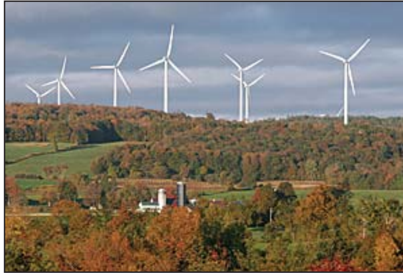
The Maple Ridge Wind Farm is a 321-megawatt project spanning the New York towns of Martinsburg, Lowville, Watson, and Harrisburg, about 75 miles northeast of Syracuse. The project produces enough electricity to power up to 160,000 average New York homes. Maple Ridge has increased the amount of wind power in New York by 600 percent. New York is a state with a 25 percent Renewable Portfolio Standard, designed to be in full effect by 2013.
