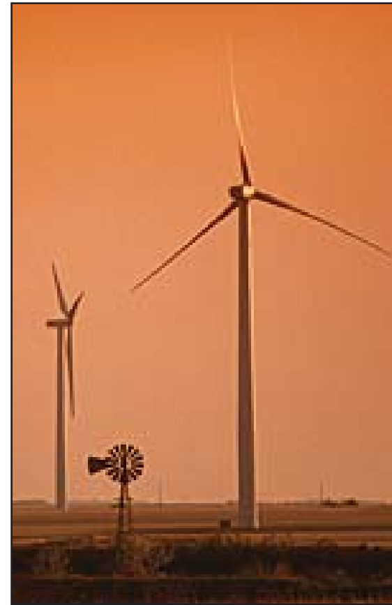
The Elk River Wind Project is a 150-megawatt wind energy project located in Butler County, Kansas.
